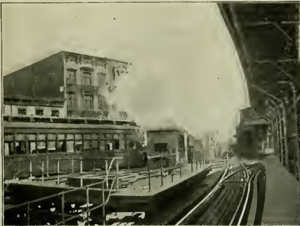
Fig. 16. CHATHAM SQUARE STATION.
